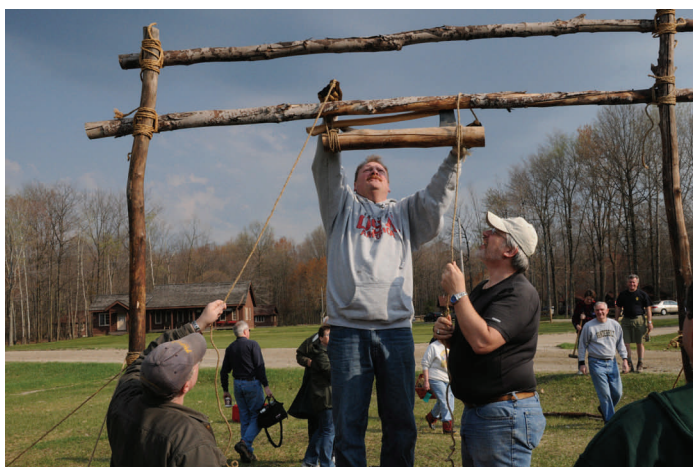
C-13-10's version of Gilwell Field Under construction
